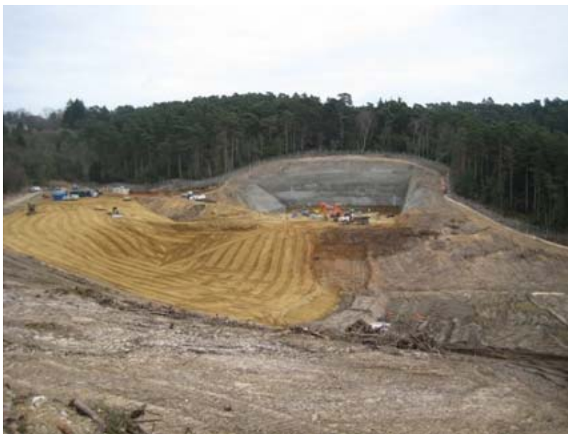
View of the south portal works for the A3 bypass and tunnel project March 2008 source HA website
